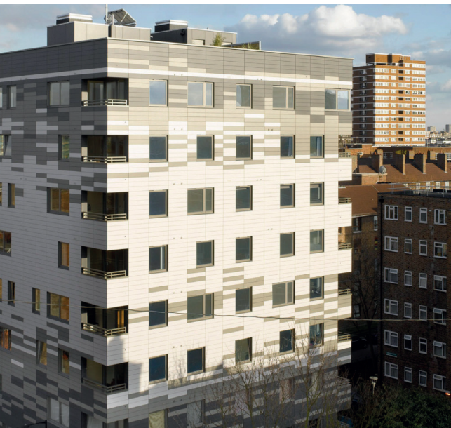
Murray Grove Residential Building, UK
